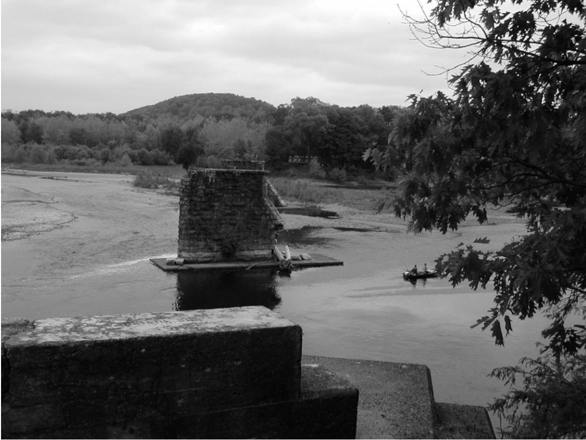
Figure 29. End of the Karamac trail. The bridge for the Lackawanna Railroad was taken out by the flood in 1955. That flood was one of the reasons for proposing the construction of the ill-fated Tocks Island dam about xxx miles upstream. Note the gravel bars in Delaware River and the higher stream terraces. The hill beyond is held up by various Upper Silurian and Lower Devonian sedimentary rocks.
