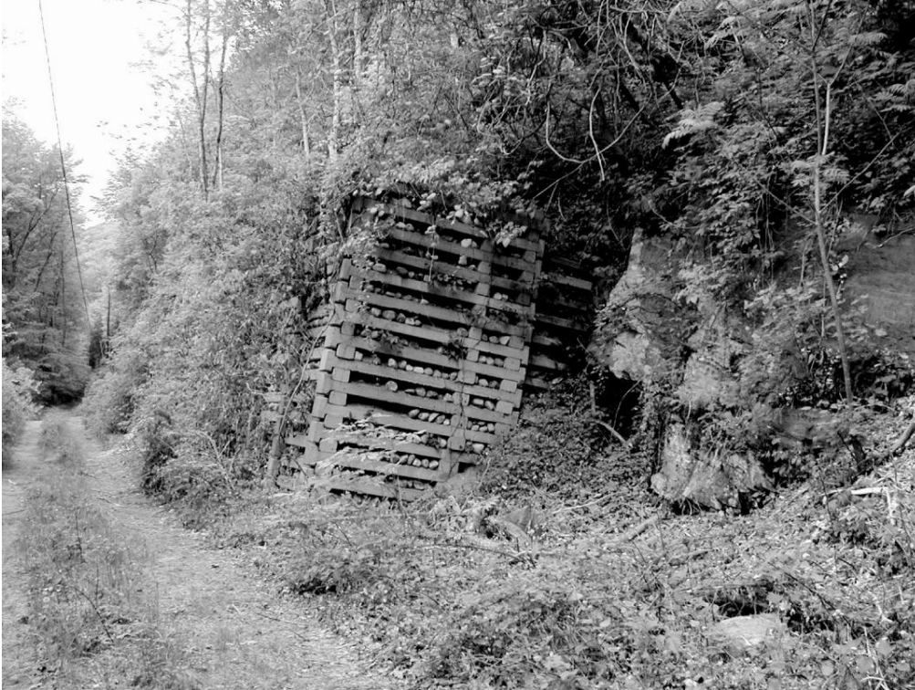
Figure 21. Concrete gabion along abandoned railroad grade below the Old Mine Road in Worthington State Park
