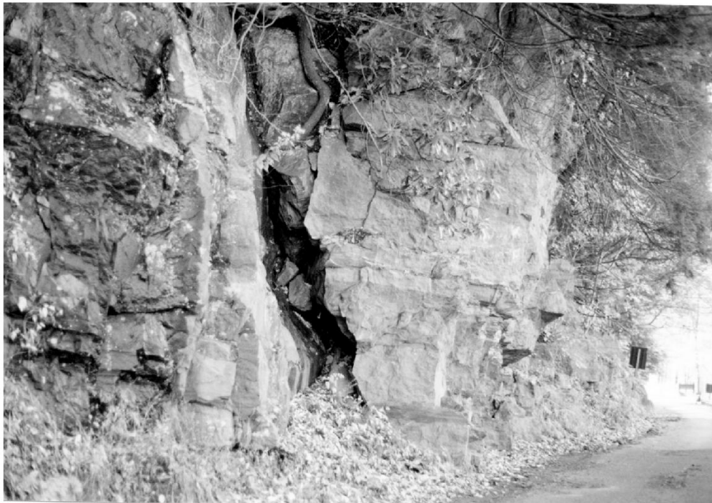
Figure 22. Irregular joints, trending along the Old Mine Road above the Karamac Trail. Boulders in the fractures are wedging the block apart, creating the potential for toppling.
